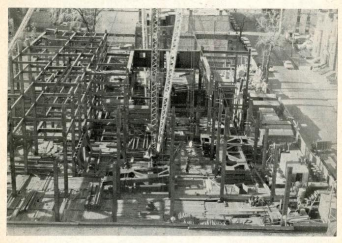
Cover photo — AERIAL VIEW, TAKEN FROM ATOP BURNSIDE STREET, OF PROGRESS IN CONSTRUCTION OF HENRY F. HALL BUILDING OF SGWU, IN NOVEMBER. MUCH OF THE STEEL FRAMEWORK IS ALREADY IN PLACE.
